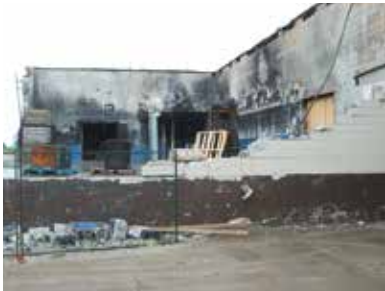
PRODUCE PLANT FIRE BEFORE
