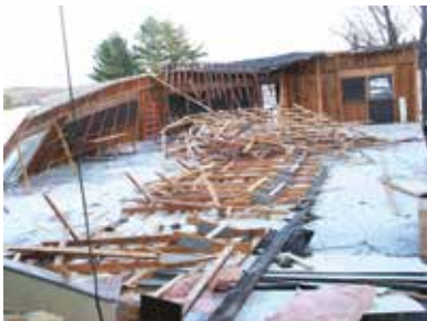
CAMP COLLAPSE BEFORE
